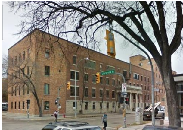
Misericordia Hospital, Winnipeg (built 1926; addition 1961): Original coal-fired T.P. Moka brick in centre; natural gas-fired T.P. Moka brick at left.
